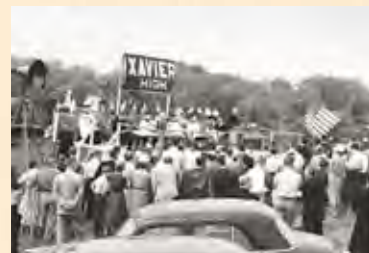
1958 groundbreaking, St. Xavier High School's new campus in Cincinnati.
