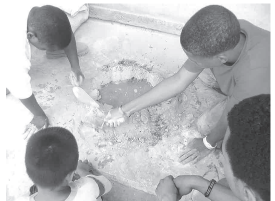
Team work: fixing a sidewalk together
